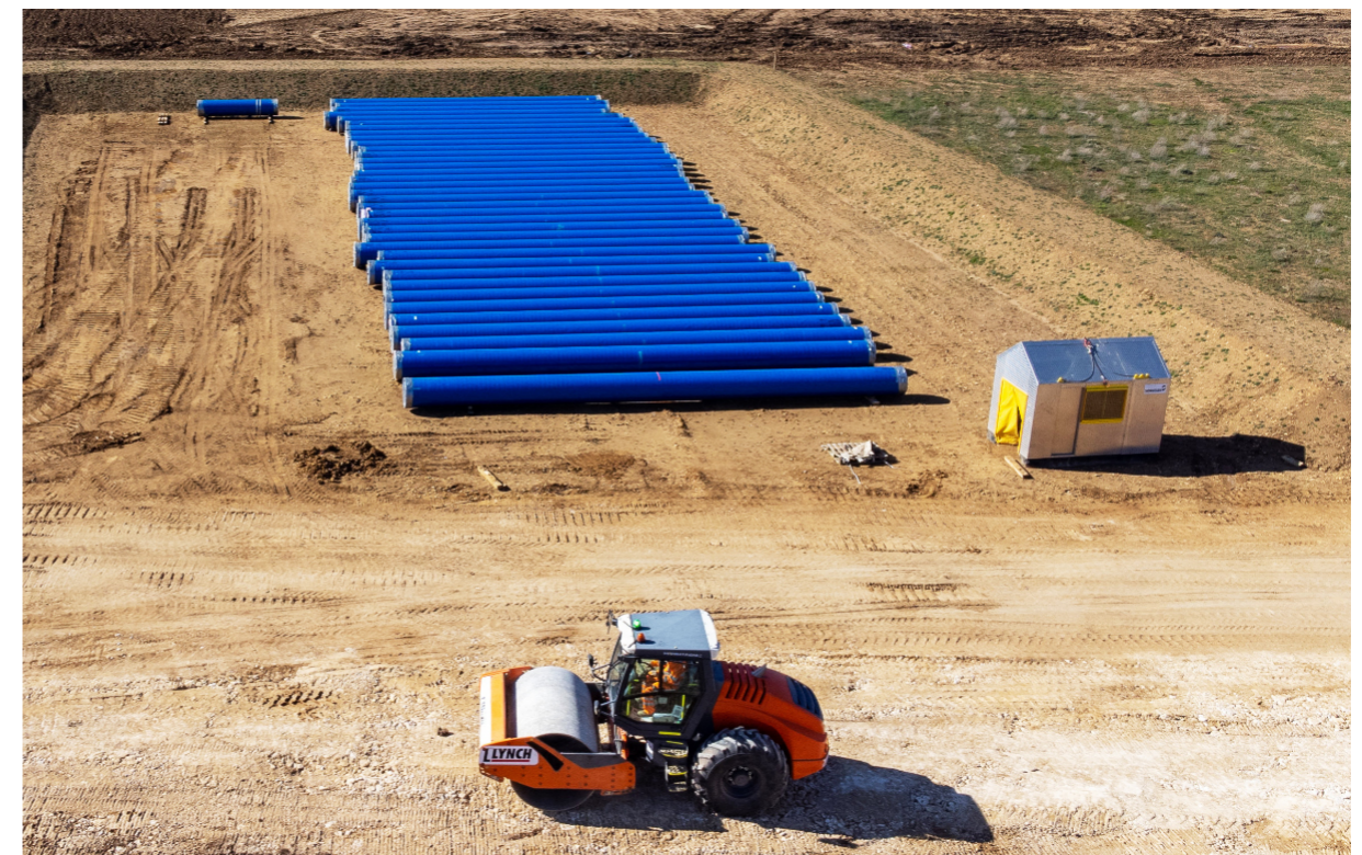
Pipeline - Anglian Water
